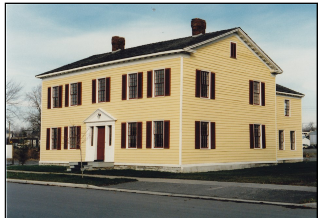
CABHC: 2023-047-02 Building after restoration, 1984
