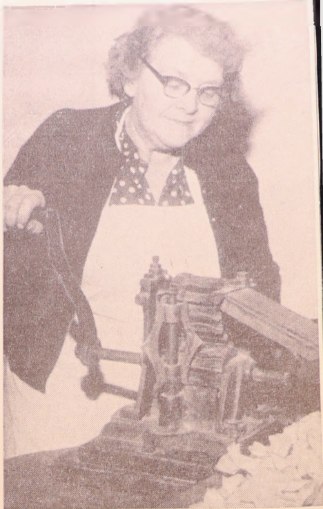
KISS CUTTER — Ruth Andrews, counter woman at Weese's Candy Store, demonstrates hand operated machine used to cut kisses. After cutting, kisses are individually hand wrapped.
