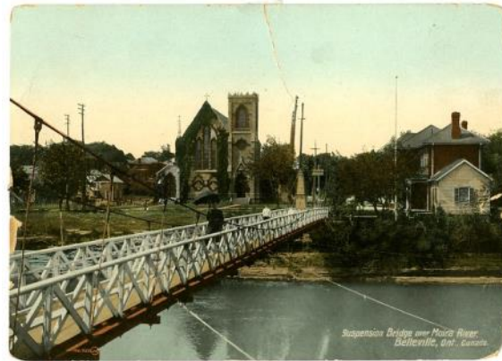
CABHC: HC00457 Valentine & Sons 'Giant' postcard showing the original suspension footbridge, commissioned in 1873 and built in 1874, c.1910
