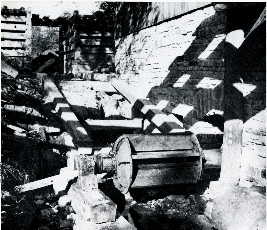
Reconstruction of the O'Hara Mill and dam has been a major project of the Authority in 1956. Seen here is the water wheel and the downstream face of the timber crib, rock filled dam. The flume and dam have now been completed and after almost fifty years of idleness the only muley saw mill in Ontario can be operated by water power.
