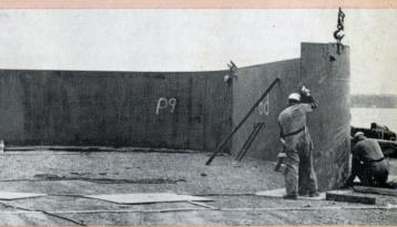
Pictured BELOW. LEFT. laborers and welders work on the scaffolding inside Caisson 10. Over 650,000 pounds of steel are required to construct the 11 caissons. The photo BELOW. RIGHT, was taken at the bridge site and shows one of the caissons being lowered into position in the Bay of Quinte. The overburden had previously been removed from the site and the bedrock excavated to a depth of one foot. Some of the piers can be seen in the background on the opposite shore.
