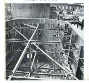
USUALLY when steel fabrication work is required on various construction projects of the McNamara organization, it is carried out at the Leaside shop of McNamara Construction Equipment Ltd. and the finished product is shipped out to the jobsite. In some cases the shop men have gone to the jobsite to carry out the fabrica-tion work, but this procedure has usually been followed only when the fabrication job has been a comparatively small operation.
