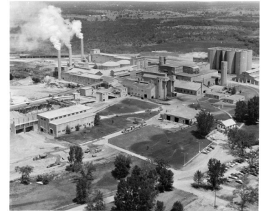
CABHC: 2017-27 Point Anne cement works, donated by the City of Belleville
