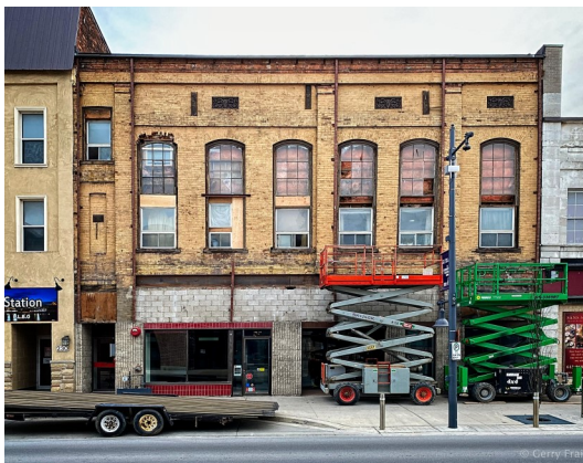
CABHC: 2021-039 232 Front Street by Gerry Fraiberg, 24 April 2021
