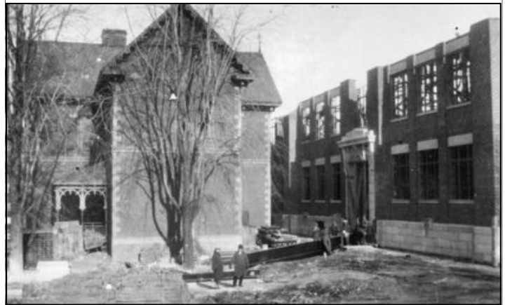
BCI under construction (at the right) Note the old Belleville high school at the left before it was torn down. Photo from Mika Collection 1927-1928
