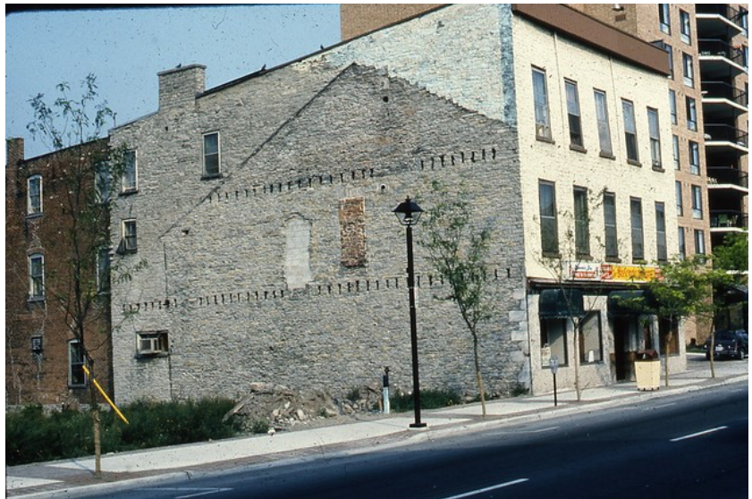
CABHC: 2021-023-161 Hotel Belvedere at 360 Front Street, Belleville, c.1987
