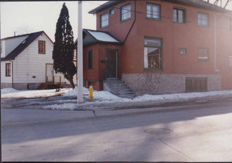
The office at 63 Moira Street West
