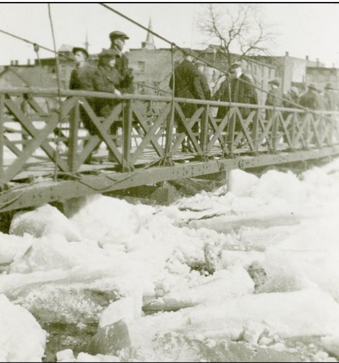
The footbridge swayed to and fro on its cable supports. HC07082D
