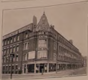
General Offices, Nottingham.
